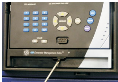
FIGURE 3-5: Press Latch to Disengage Handle
